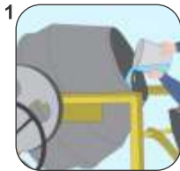
1 Add 70% of water to concrete mixer.
